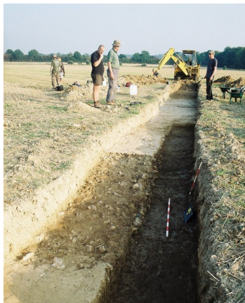
5: TT2 during excavation with JCB
