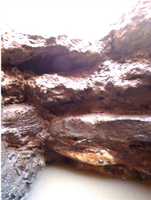
6.9: The interior of wall forming the well
