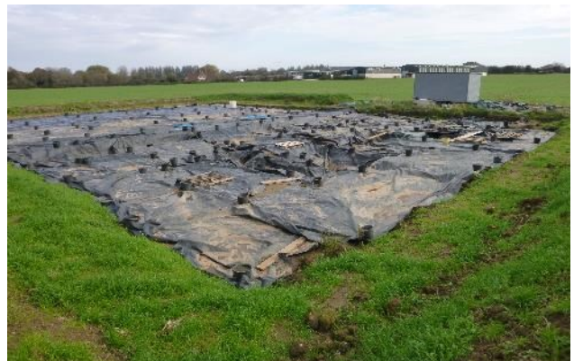
8.31: Trench covered and site cabin installed
