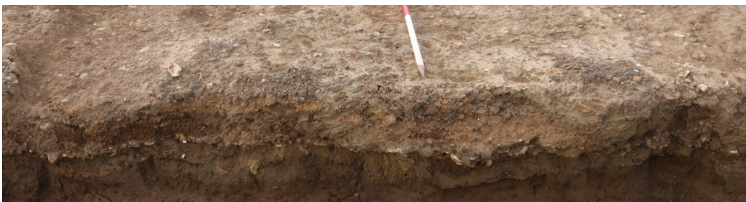
7.16: The north facing section of Slot 12 showing the road structure
