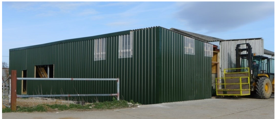
5.1: the facilities block under construction in May 2015
