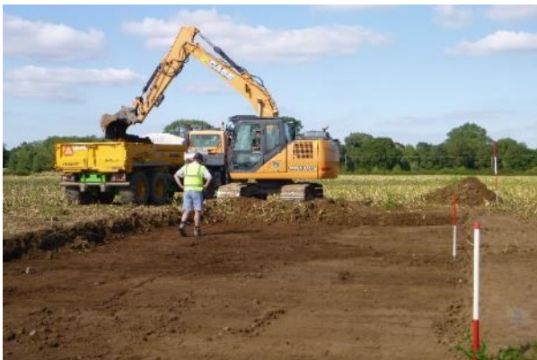
8.30: Removing overburden from the new area
