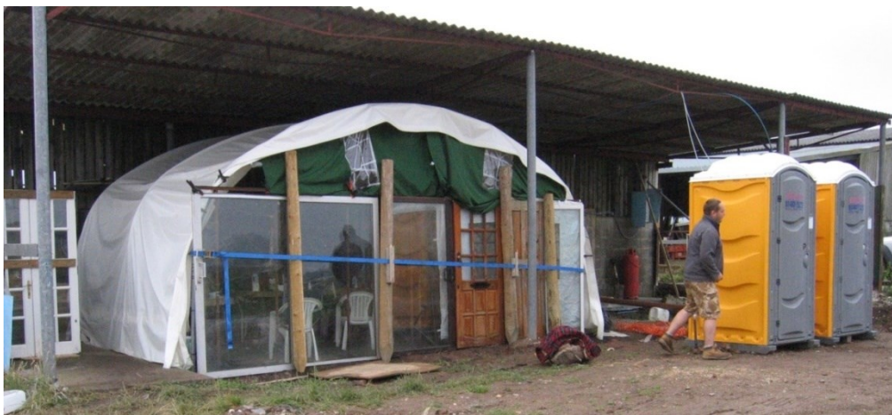
5.2: The make-shift 'refectory' and portable facilities of 2014, housed in the open shed that was the basis of the new HQ building
