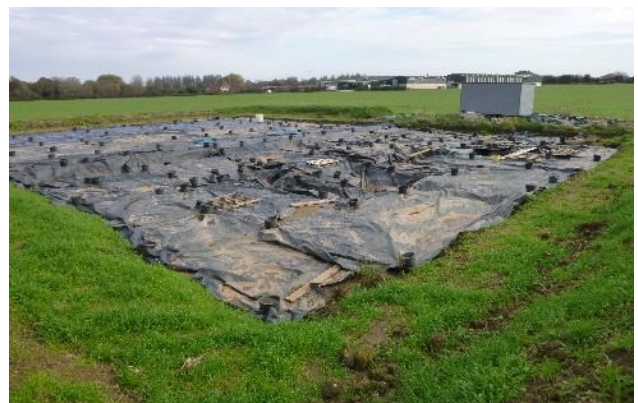
8.31: Trench covered and site cabin installed
